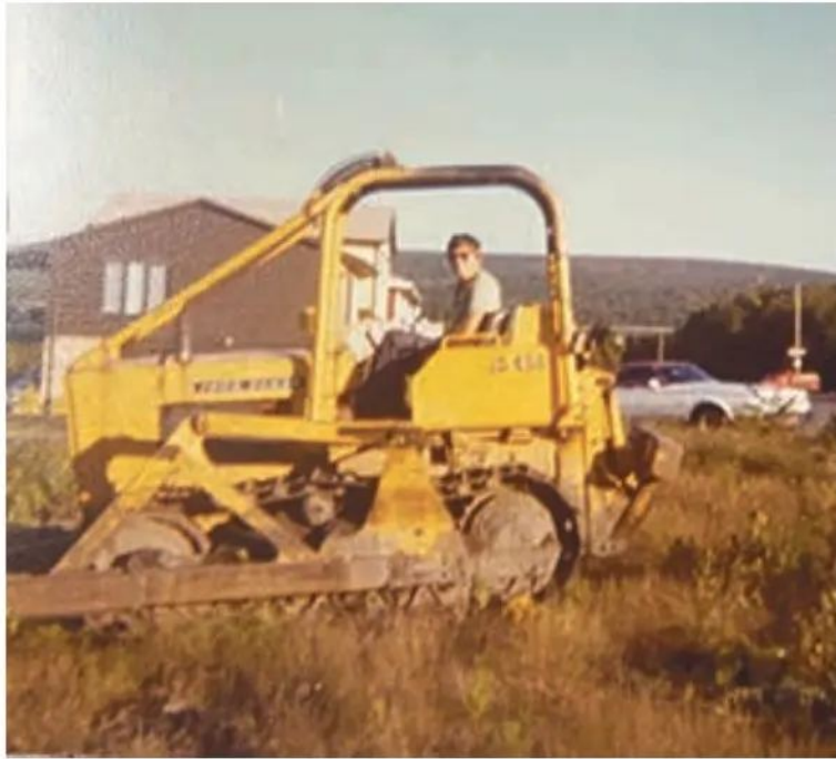
Tom Swinick is shown on a bulldozer in his development back in 1979.
